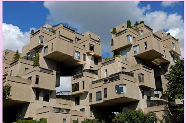
Habitat 67 on St. Helene Island, Montreal, Quebec, Canada
